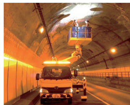
Fig.1. Inspecting the walls inside a tunnel from the deck of an inspection vehicle
