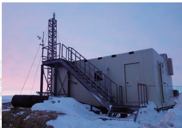
Fig.2. The atmospheric observation room for clean air (AOH) at the Syowa Station, where aerosol observations are carried out. Air is drawn in from the top parts of the tower on the left.
